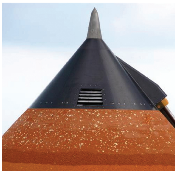
Figure 7-12. STS-117 ET hail damage, February 2007.
