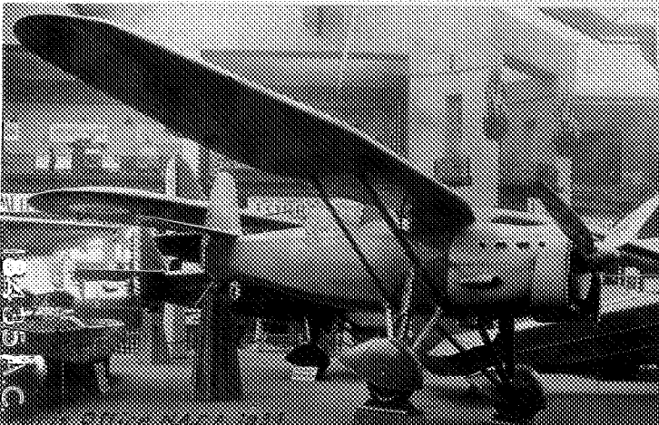
Figure 14.- Mureaux 180 C.2 Two seat fighter. (890 hp. Hispano-Suiza engine. 20 mm cannon)
