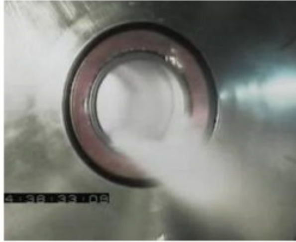
Figure 5. Condensation water discharge from facility prior to installation of extraction flange.
