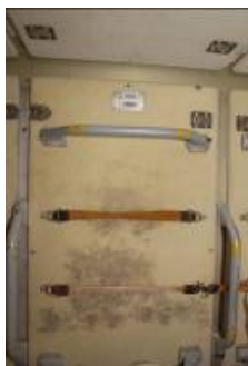
ISS010E11563 — An example of microbial contamination that developed on interior panel 406 aboard ISS. Following workouts, the crewmembers placed their clothes on this panel to dry out. Attempts to clean this panel with supplies aboard ISS failed, and the panel had to be replaced.
