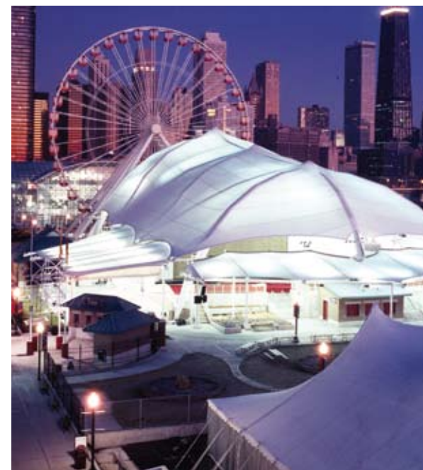
Apollo-era space suit fabric proved useful for designing visually intriguing, large-scale, permanent tensile fabric roofs, like the one seen here at Chicago's Navy Pier.
