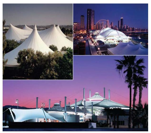
Fabric (a blend of GORE-TEX, Kevlar, and Nomex—all private industry inventions) in its ITMG instead of the PTFE fiberglass fabric, that original innovation has gone on to become a unique component of an unrelated, terrestrial field: architecture.
