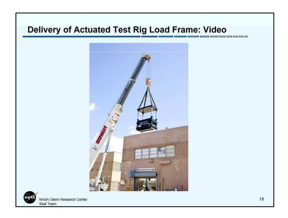
The sheer size of the new load frame required a creative delivery approach as it would not easily fit through the front garage door. The Space Exploration Seal System Lab's roof hatch is removable allowing riggers to lower it through the roof as shown in this still frame from the movie shown during the workshop.
