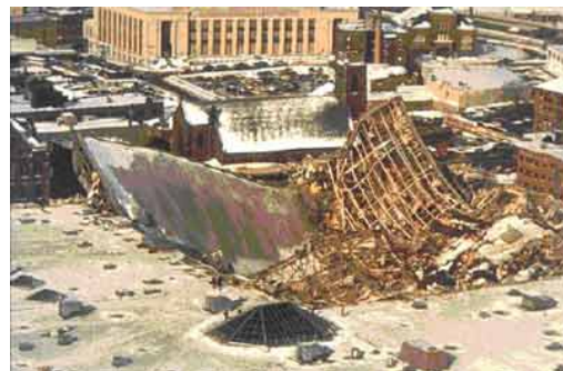
Figure 2. Hartford arena roof collapse. *
