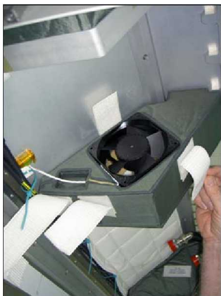
Figure 11. Intake fan soft captured in foam abatement.
