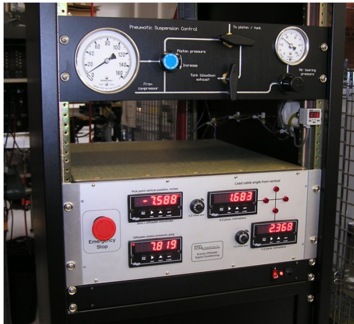
Figure 9: Piston pressure in psig (lower left) and carriage position from center in inches (upper left) on the control console. Tip-tilt sensor outputs in milliradians are displayed on the other two readouts.
