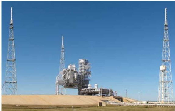
Figure 7. The single lightning mast atop the fixed service structure (FSS) at LC 39B (top) was replaced by a trio of towers (bottom).
