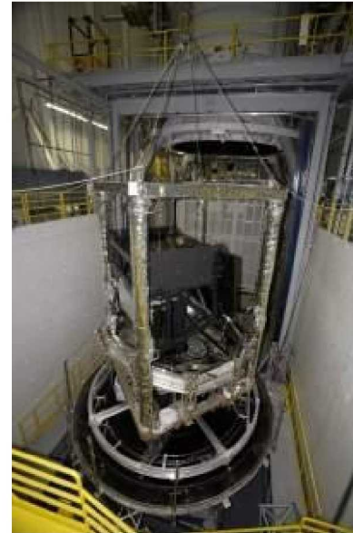
Installation on Chamber Lid
