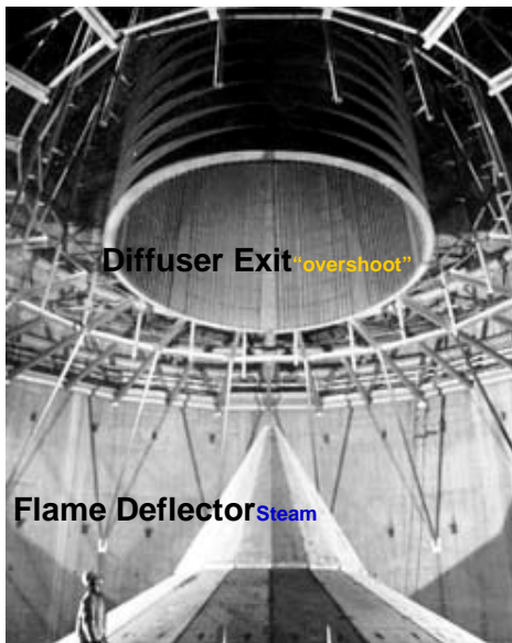
Figure 23. S-IVB 'Battleship' Stage Installation Details in J-4 Test Cell
