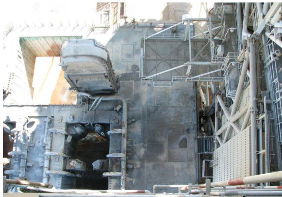
Figure 13. Ares I-X caused more damage to Launch Complex 39B than a Shuttle flight.
