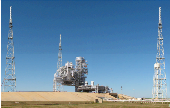
Figure 12. The single lightning mast atop the fixed service structure (FSS) at LC 39B (top) was replaced by a trio of towers (bottom).
