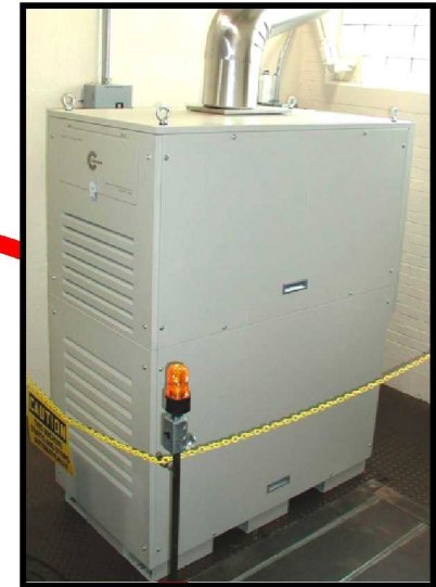
Capstone MicroTurbine proof-of-concept & environmental durability test facility
