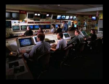
In 1990 a WDPF (Westinghouse Distributed Process Family) control system was installed in PSL.
