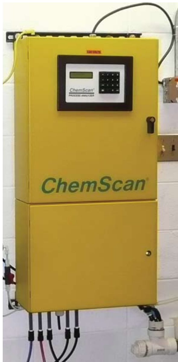
The ChemScan analyzer ties directly into a treatment facility's control system, minimizing the need for operator intervention.
