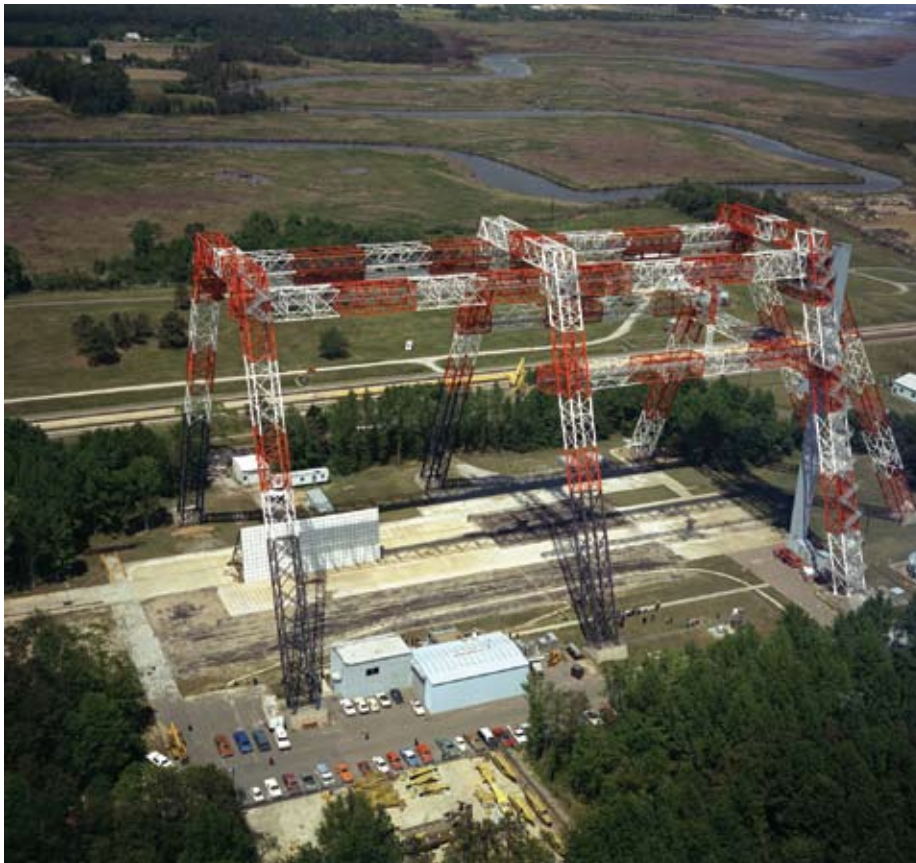
Originally built to allow Apollo astronauts to practice landing on the Moon, this 240-foot-high gantry (left) is now Langley Research Center's Landing and Impact Research Facility. Crashworthiness testing at the facility (right) allowed Cirrus Design Corporation to improve survivability during stall/spin impacts.
