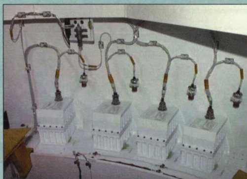
Four EDAS units were installed in the forward skirt on the right-hand booster for shuttle mission STS-91 in June 1998.
