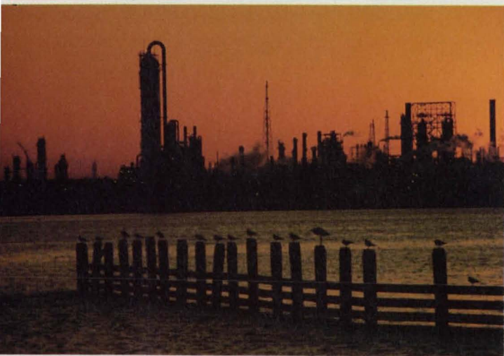
A chemical plant in Texas City
