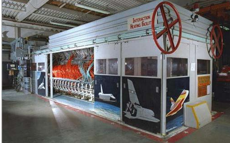
Figure F-2. Ames Interaction Heating Facility (IHF).
