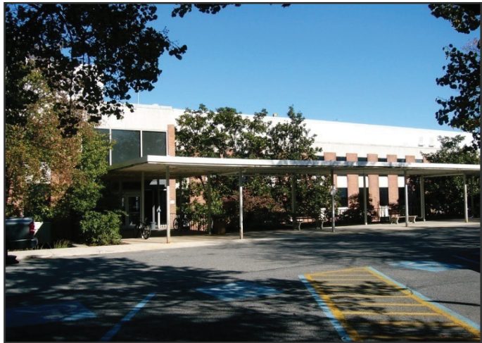
Building 21 main entrance. Although B21 does not look as though it has changed much from the outside, the renovations inside will make a significant difference to the efficient functioning of HSD.
