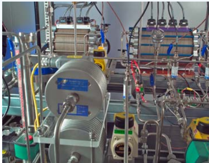
Integrated system test set up of closed loop hydrogen oxygen regenerative fuel cell system
