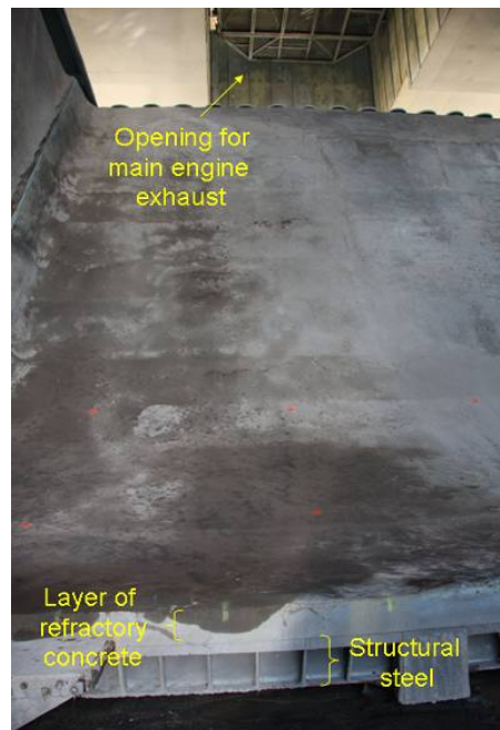
Figure 4. Magnified View of LC-39A Flame Deflector
