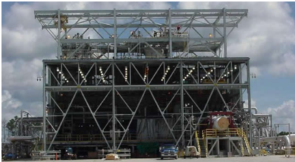
Figure 40. Stennis E-1 Flame Deflector
