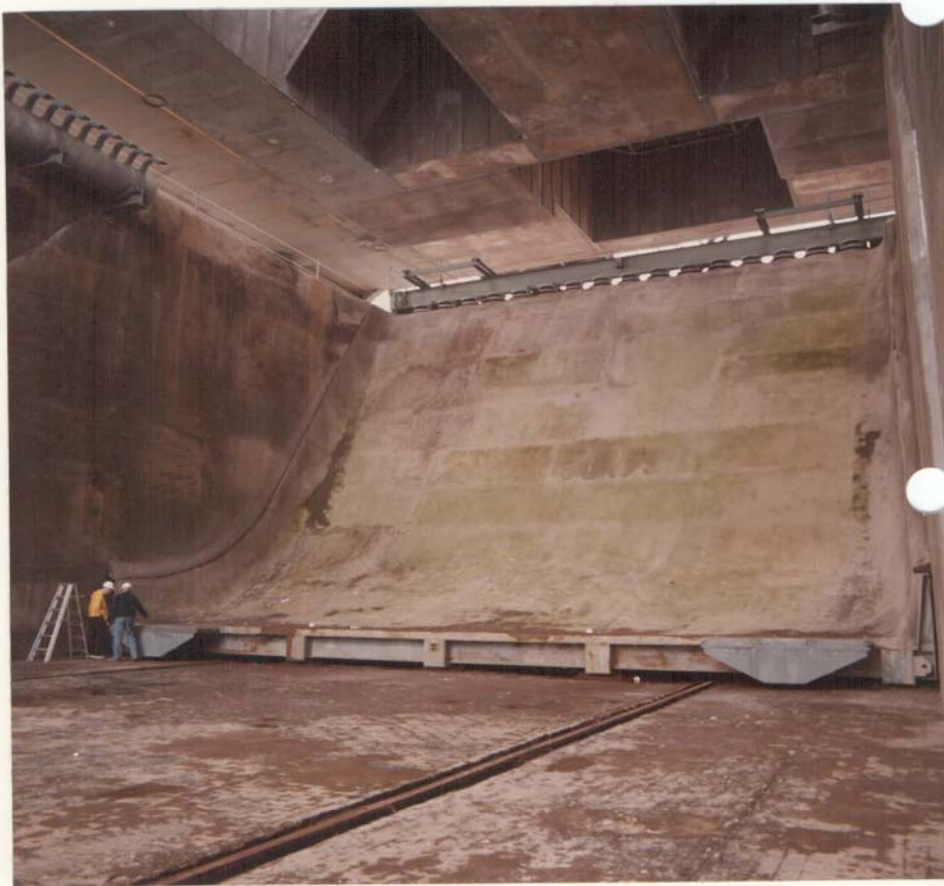
FIGURE 1 FLAME TRENCH, SHOWING TEST FRAMES AT BOTTOM OF FLAME DEFLECTOR
