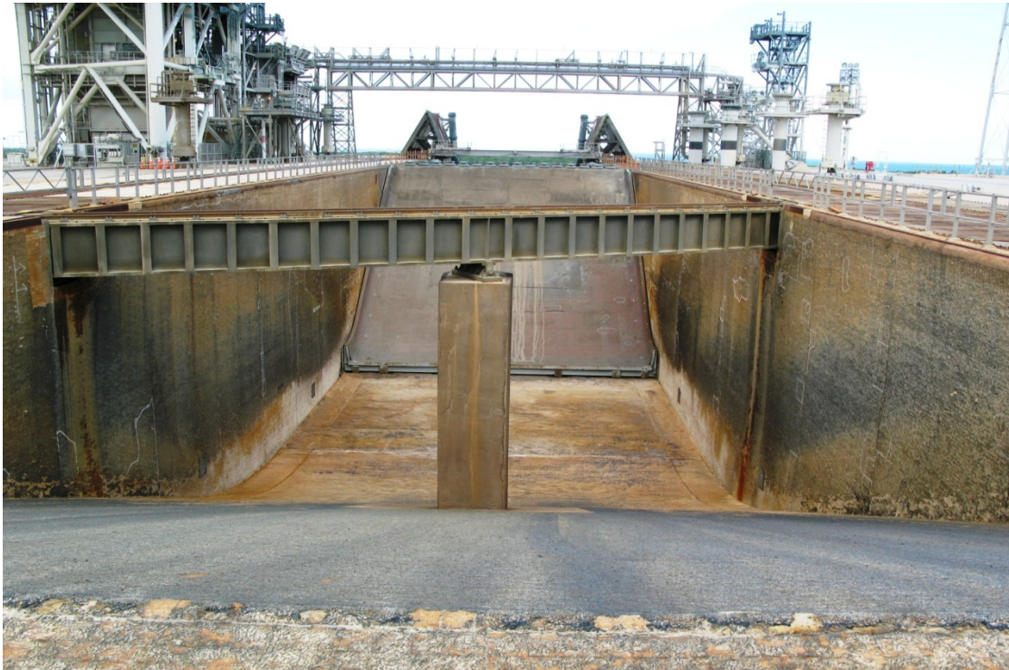
Figure 5. SSME Flame Trench and Deflector
