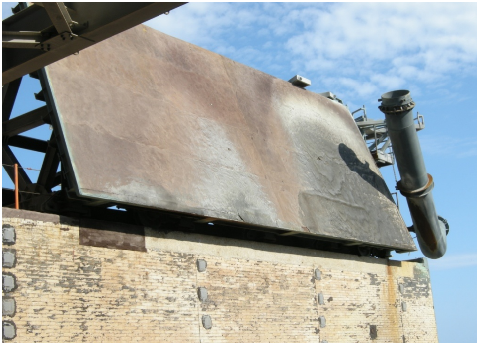
Figure 7. Side Flame Deflector
