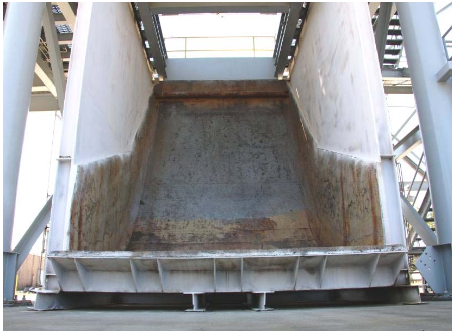
Figure 42. Stennis Space Center E-2 2 Vertical Test Flame Duct
