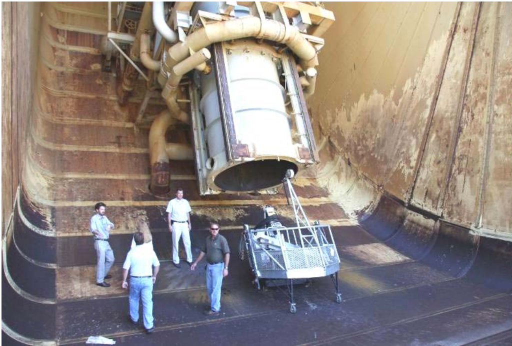
Figure 37. View of the A-2 Flame Duct and Diffuser
