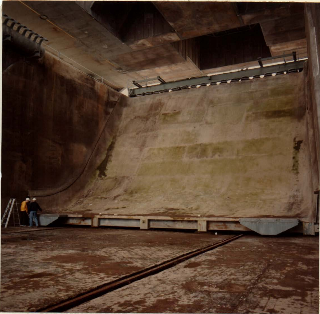
FIGURE 3. SRB FLAME DEFLECTOR AND TEST FRAMES.
