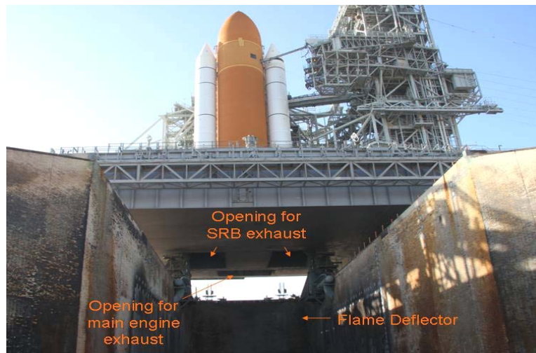
Figure 3. Openings for Flames From the Main Engine and SRBs
