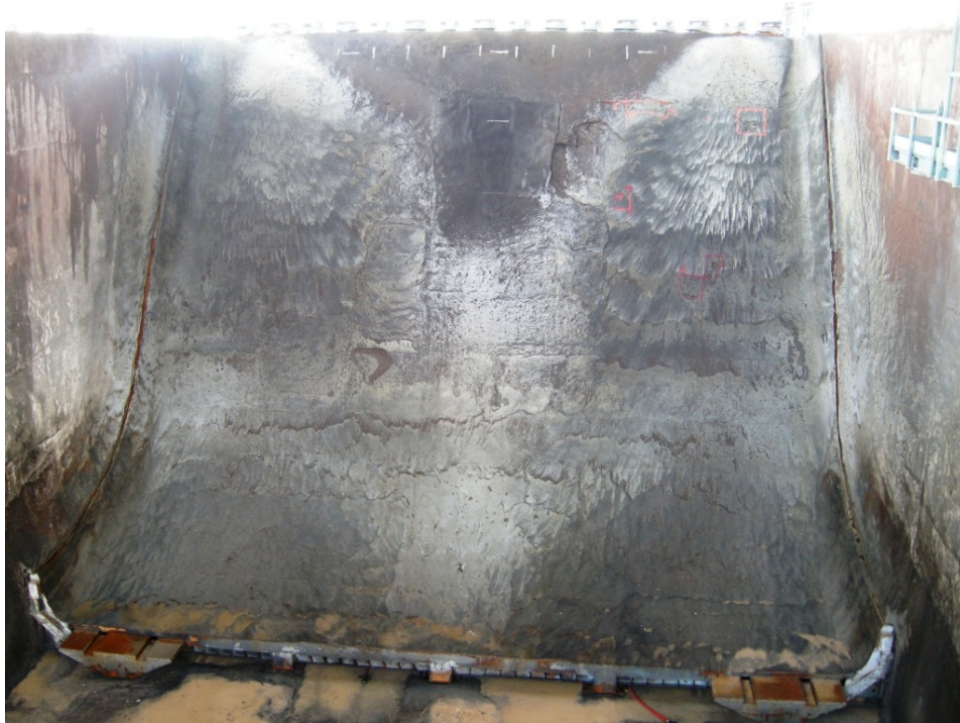
Figure 6. SRB Main Flame Deflector
