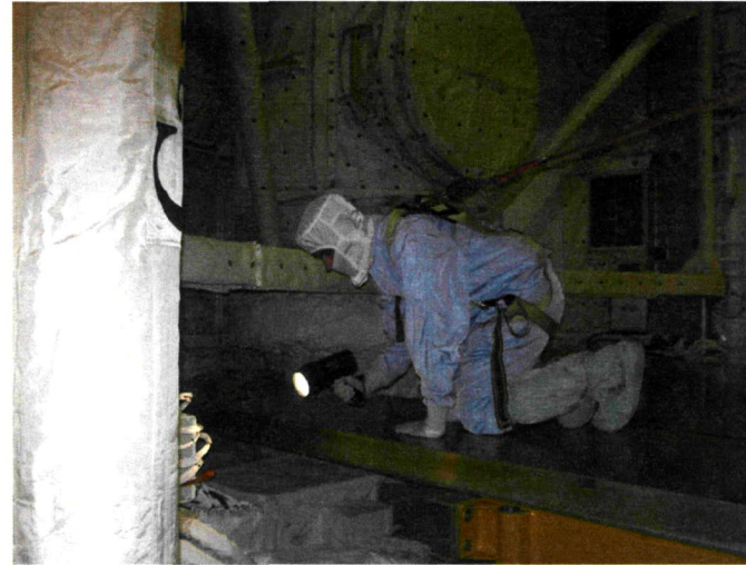
Inspection and Closeout
