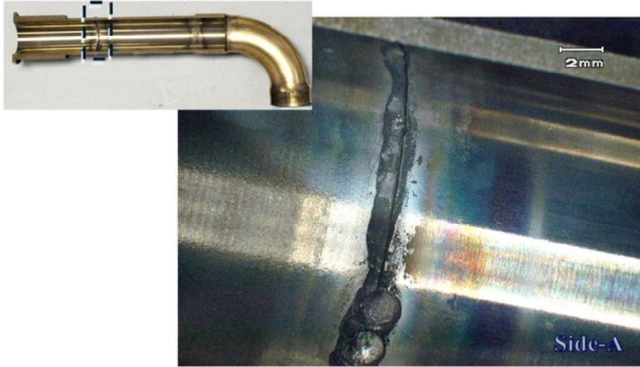
Figure 6.—Internal view of connecting pipe butt weld showing incomplete filling of the joint and the presence of hot spot metal nugs on the inside surface of the pipe.
