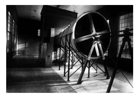
Langley Laboratory's first wind tunnel, a replica of a 10-year-old British design, became operational in June 1920. (NASA Headquarters—Greatest Images of NASA [NASA HQ GRIN].)
