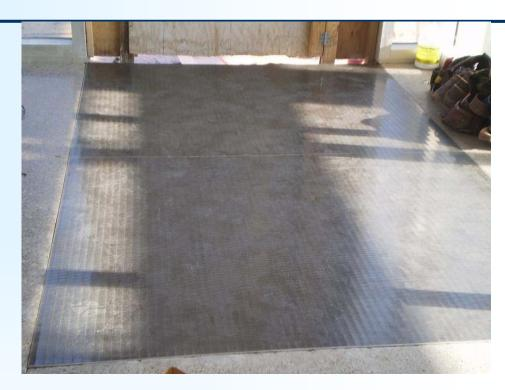
Each office has an eraser board built into the wall •Entry mats at the two main entrances have a cavity below them that capture particles from the shoes of incoming occupants, minimizing the particles floating around the building
