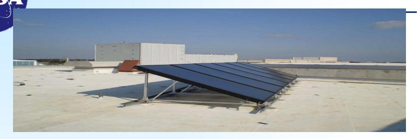
•The building utilizes a solar water heating system that transmits heat generated from roof mounted solar panels into the building's hot water system, reducing the buildings foreign energy consumption.
