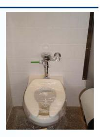
•Plumbing fixtures were selected based on their water savings potential through the use of waterless urinals, dual flush flushometers for the water closets and 0.5 GPM electronic faucets with controls to operate in 10 second durations
