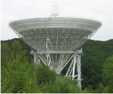
Figure 1. Effelsberg 100-m telescope with primary focus cabin at the top.
