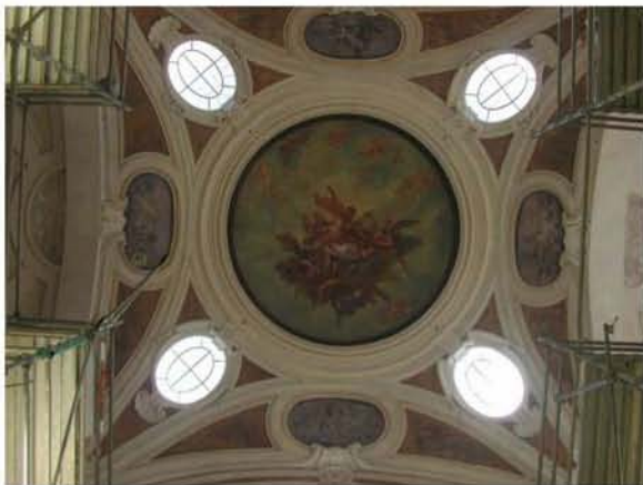
Turin, Chiesa della Misericordia, before and after restoration
