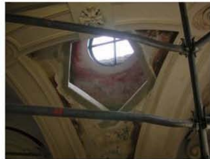
Several stages of construction: application of towels for ripping, tearing and opening of the "pentagon" after "ripped" the frescoes
