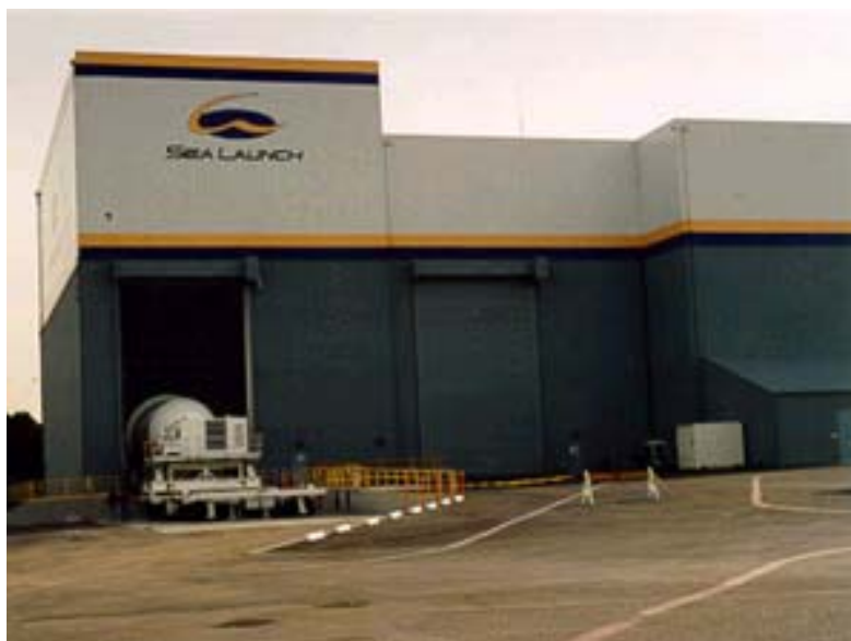
Figure B.9-3 Sea Launch Base Facilities
