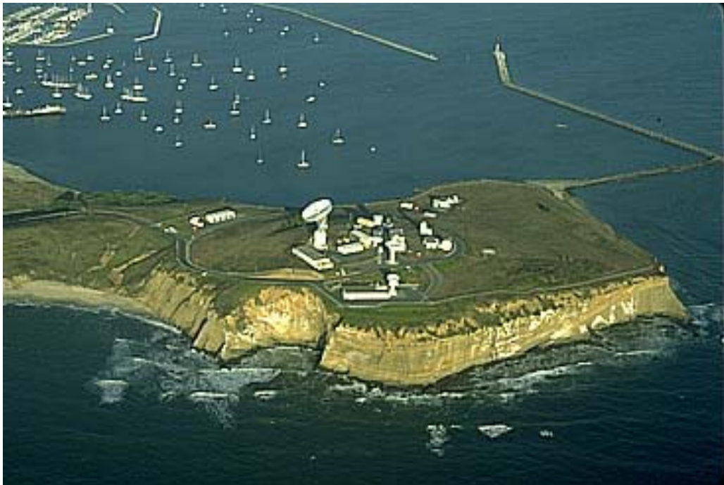
Figure B.3-9 Pillar Point Instrumentation Site
