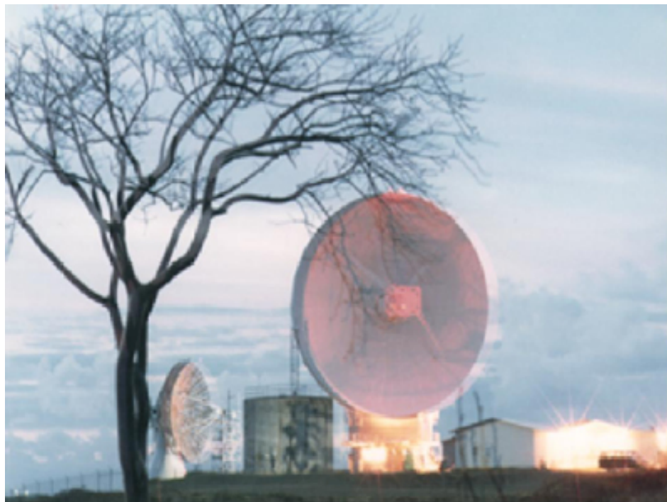
Figure B.1-27 Antigua 91.14 – MIPIR (front) (Rear dish is TAA-8 Telemetry antenna)
