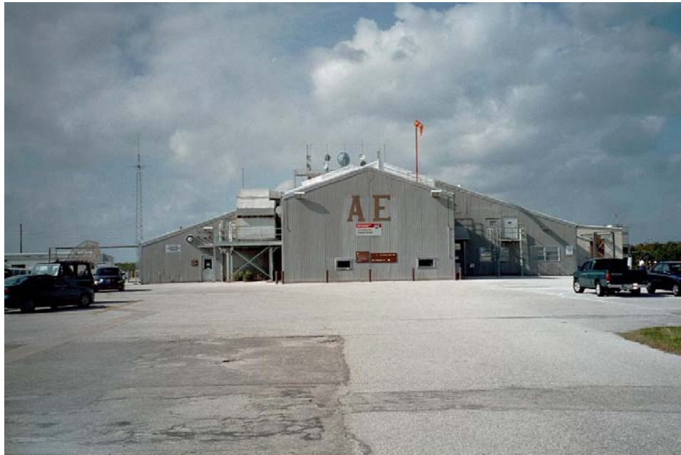
Figure B.2-30 NASA's Hangar AE on Cape Canaveral Air Station
