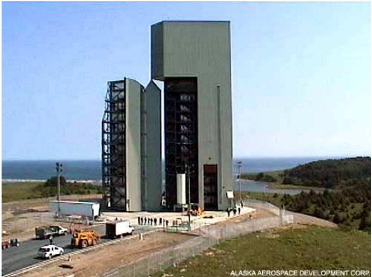
Figure B.6-6 Launch Pad 1 With Enclosure
