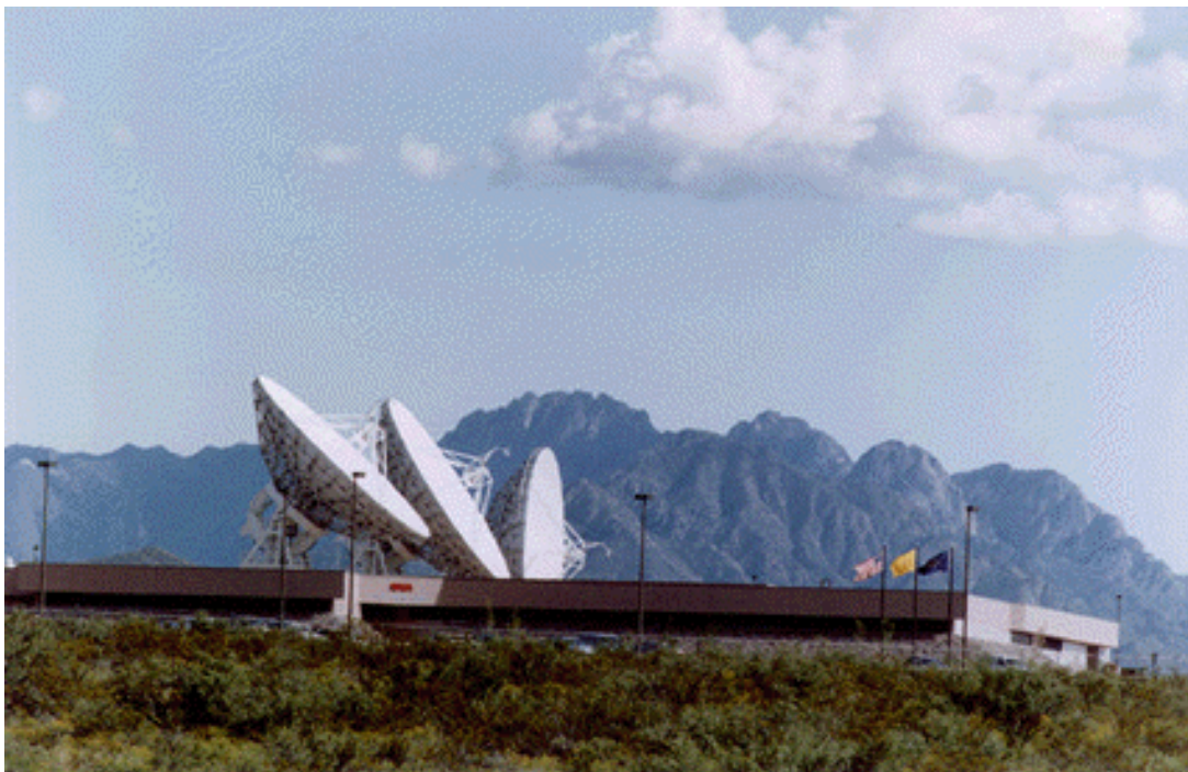
Figure B.2-28 Secondary TDRS Ground Terminal (STGT)
