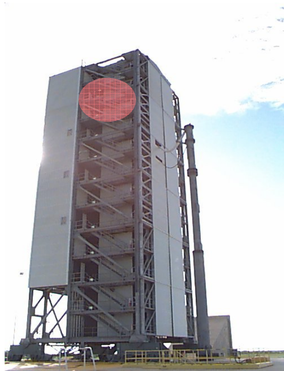
Figure 7-4 LCX-46 Service Tower
