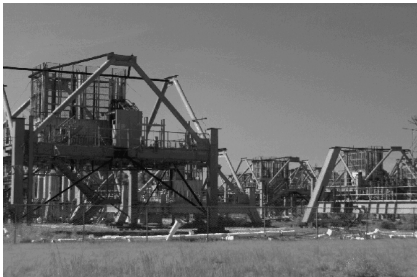
Figure B.2-41 Apollo Umbilical Towers In Storage At KSC
