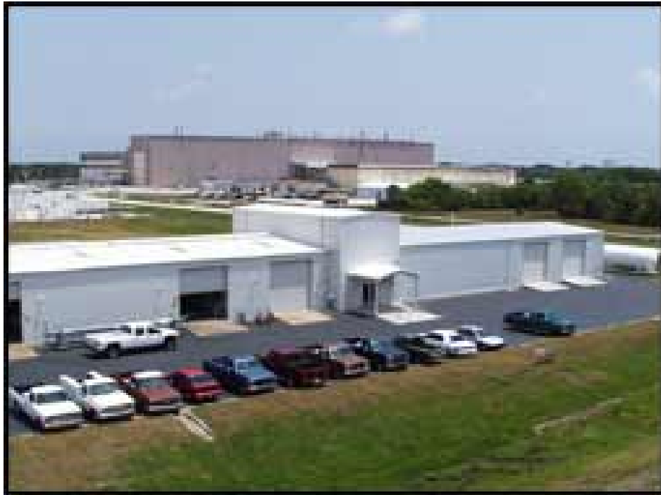
Figure B.2-34 KSC Cryogenics Test Facility
