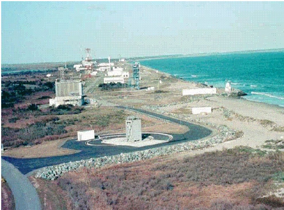
Figure 3-18 Wallops Island Launch Facilities
