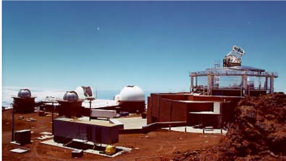
Figure B.11-5 Maui Space Surveillance Site (close up)
