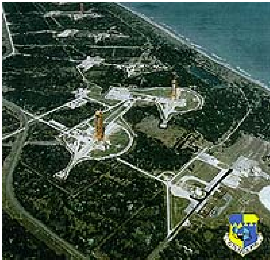
Figure B.1-14 Cape Launch Complexes in 1990's
