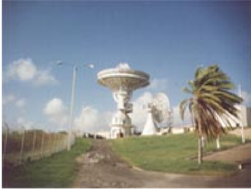
Figure B.1-18 Antigua Telemetry Antennas
