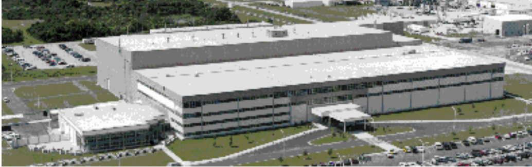
Figure B.2-47 Space Station Process Facility (SSPF)
