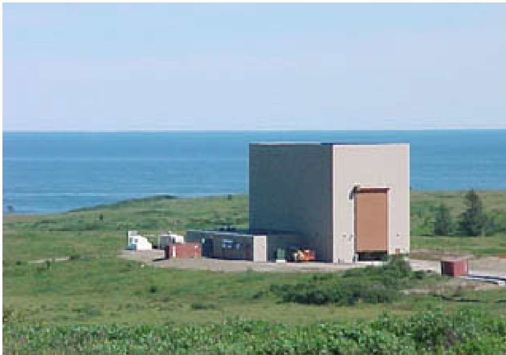
Figure B.6-3 Payload Processing Facility
