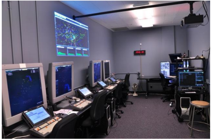
Figure 16. Air traffic control room in the AOL
