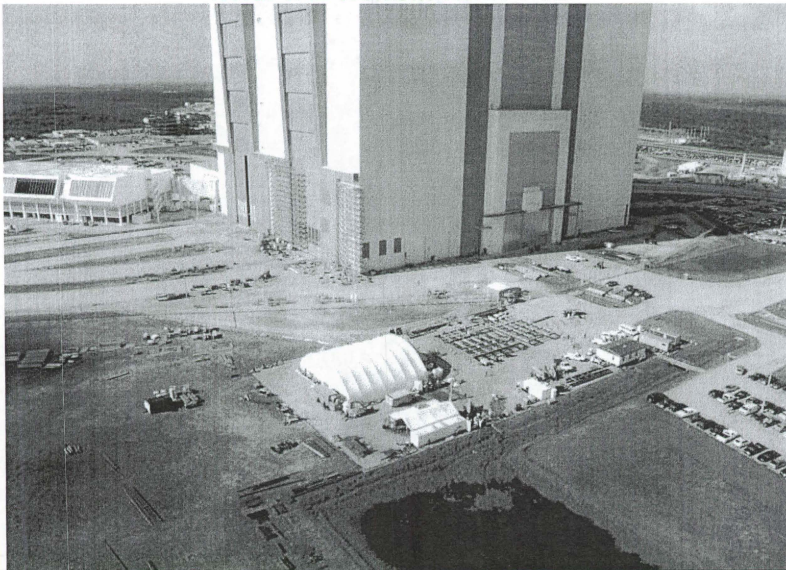
North VAB Worksite Aerial View
