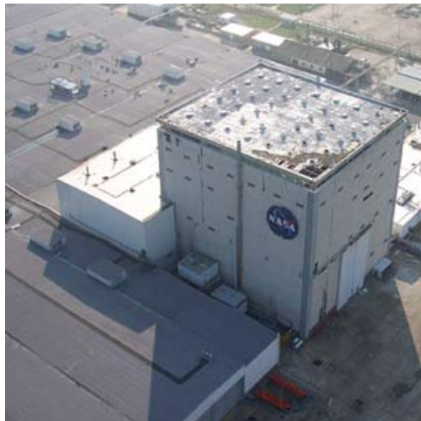
Hurricane Katrina caused damage to NASA facilities, including Stennis Space Center and the Michoud Assembly Facility, pictured here.
