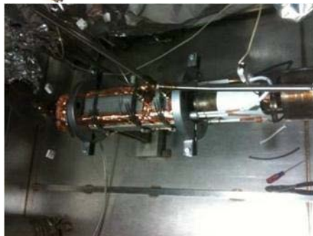
Enhanced heating assembly ready for application of insulation
