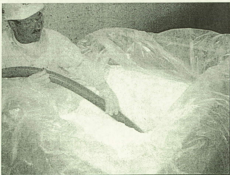
Microspheres being transferred (with suction hose) into the cryogenic tank.
