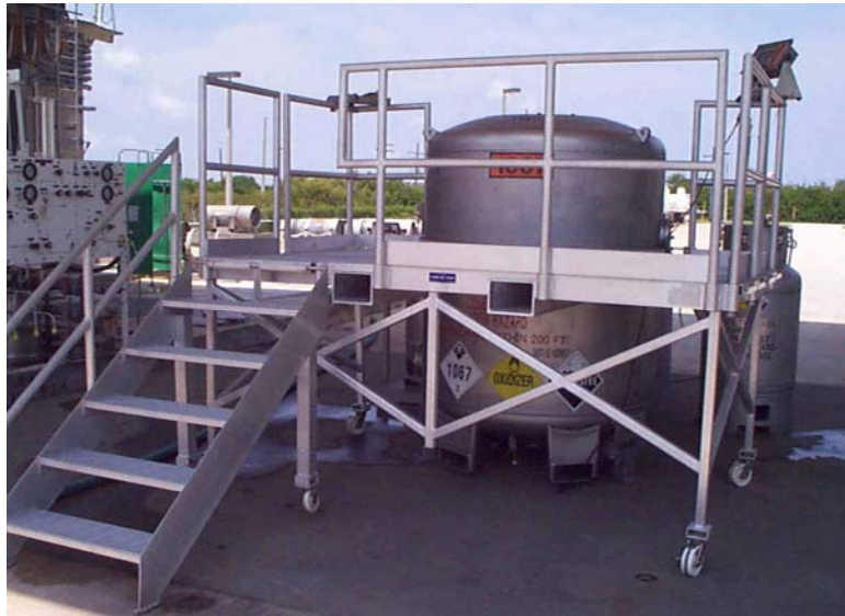
GPTU fluid system access is supported with roll-around platform and stairs
