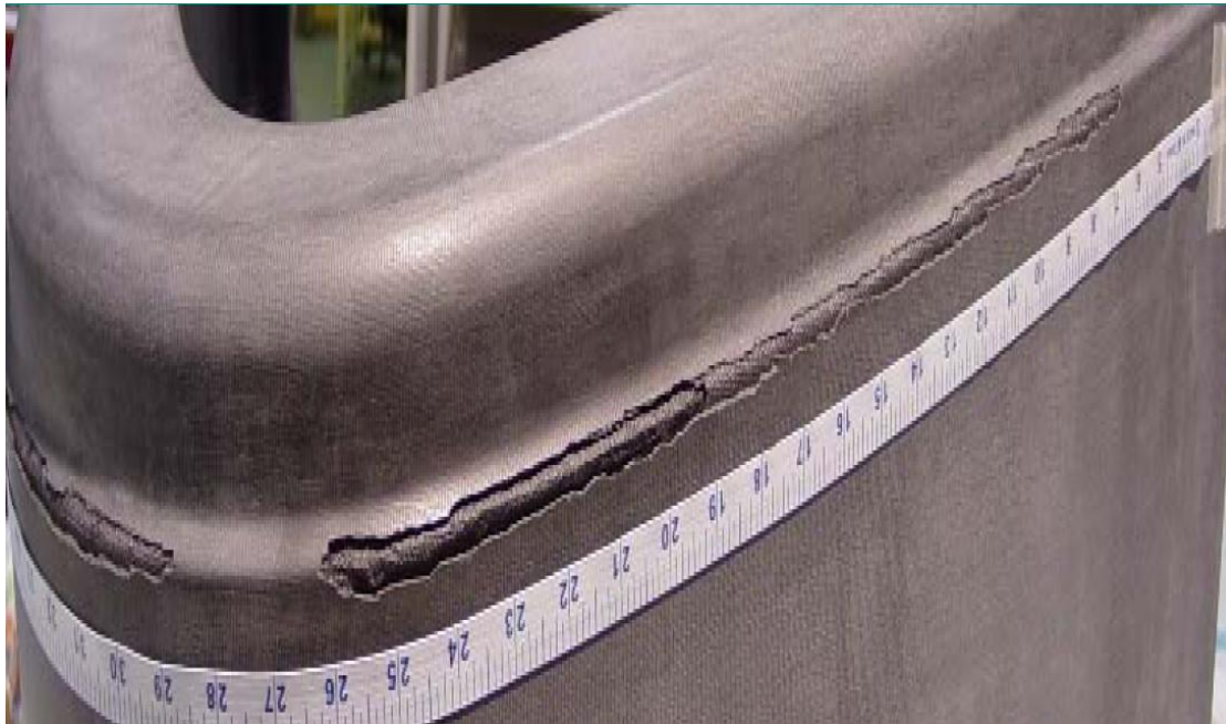
Fig. 3 Photograph of panel 8R showing slip-side joggle that had coating removed with dental pick during repair process.
