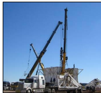
Drilling Rig Assembly
