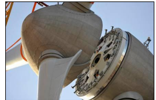
Crane Hoisting Propeller onto Windmill
