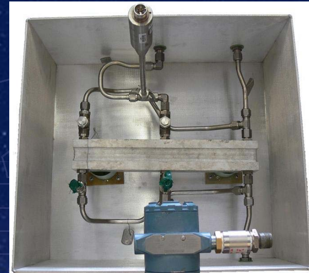
Heat exchanger being readied for upcoming LH 2 test.
