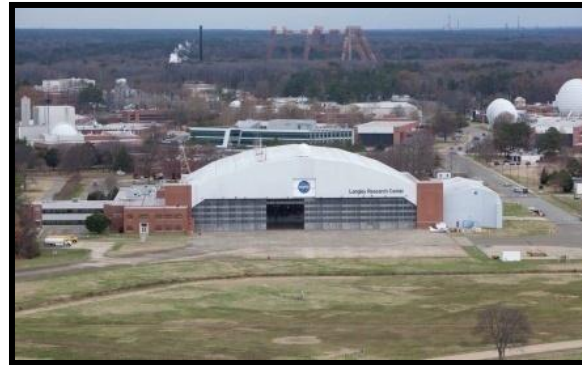
Hangar and aircraft fuel storage (multiple functions in B1244 unrelated to aircraft operations)
