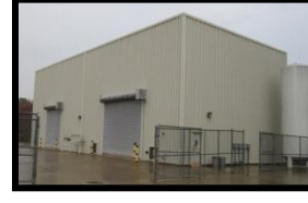
Thermal Structures Lab (B1256C)
