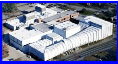
14- by 22-Foot Subsonic Tunnel Subsonic, Alternate Uses B1212
