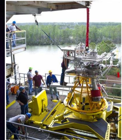
Installing the J-2X powerpack in test stand at SSC.
