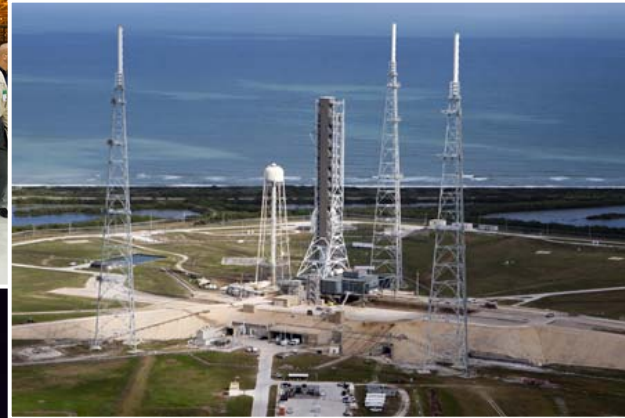
KSC is preparing Launch Complex 39B for SLS/Orion operations, 2012.
