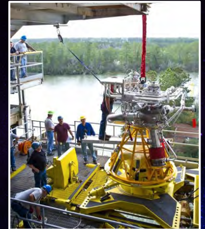
Installing the J-2X powerpack in test stand at SSC.
