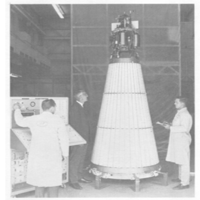
Figure II-92. SNAP 10A Flight System
