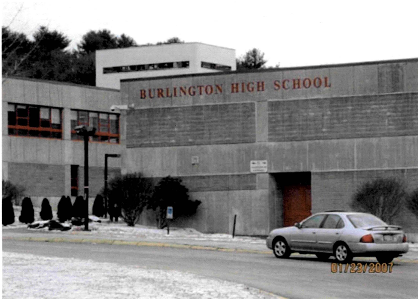
Burlington High School, Burlington, Massachusetts, 2006 Masonry Caulk 106,611ppm Arochlor 1260
