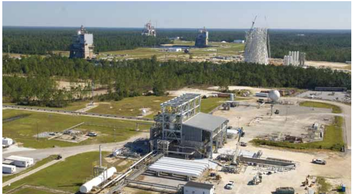
Stennis Space Center is the premier rocket engine test facility in the Nation. All three of the Center's test complexes—the E Test Complex (foreground), the three A Test Complex stands (middle) and the B Test Complex (back) are visible in this aerial photo.
