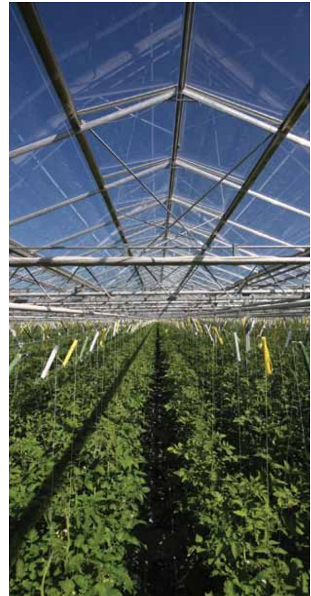
GreenField Solar's concentrators produce an excess of thermal heat that can be used for secondary purposes, such as heating nearby buildings or even greenhouses.
