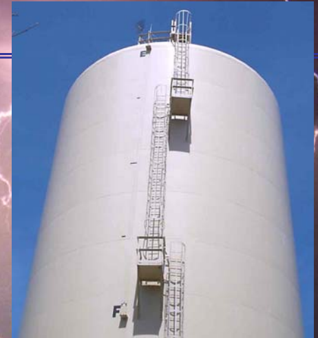
Water tower (Keel)
