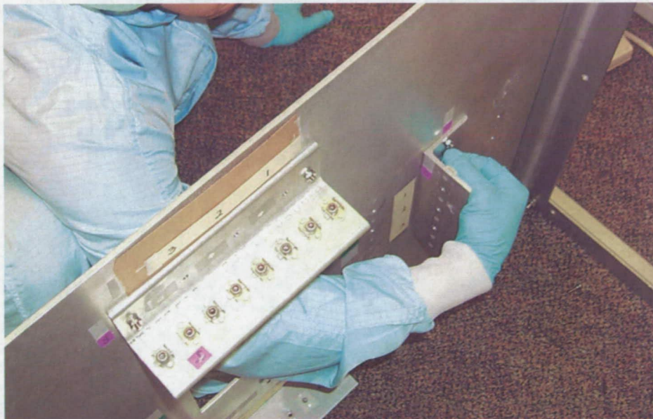
Figure 17. Technician installing screw into hole in group 6
