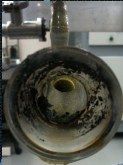
Sublimator outlet line blockage
