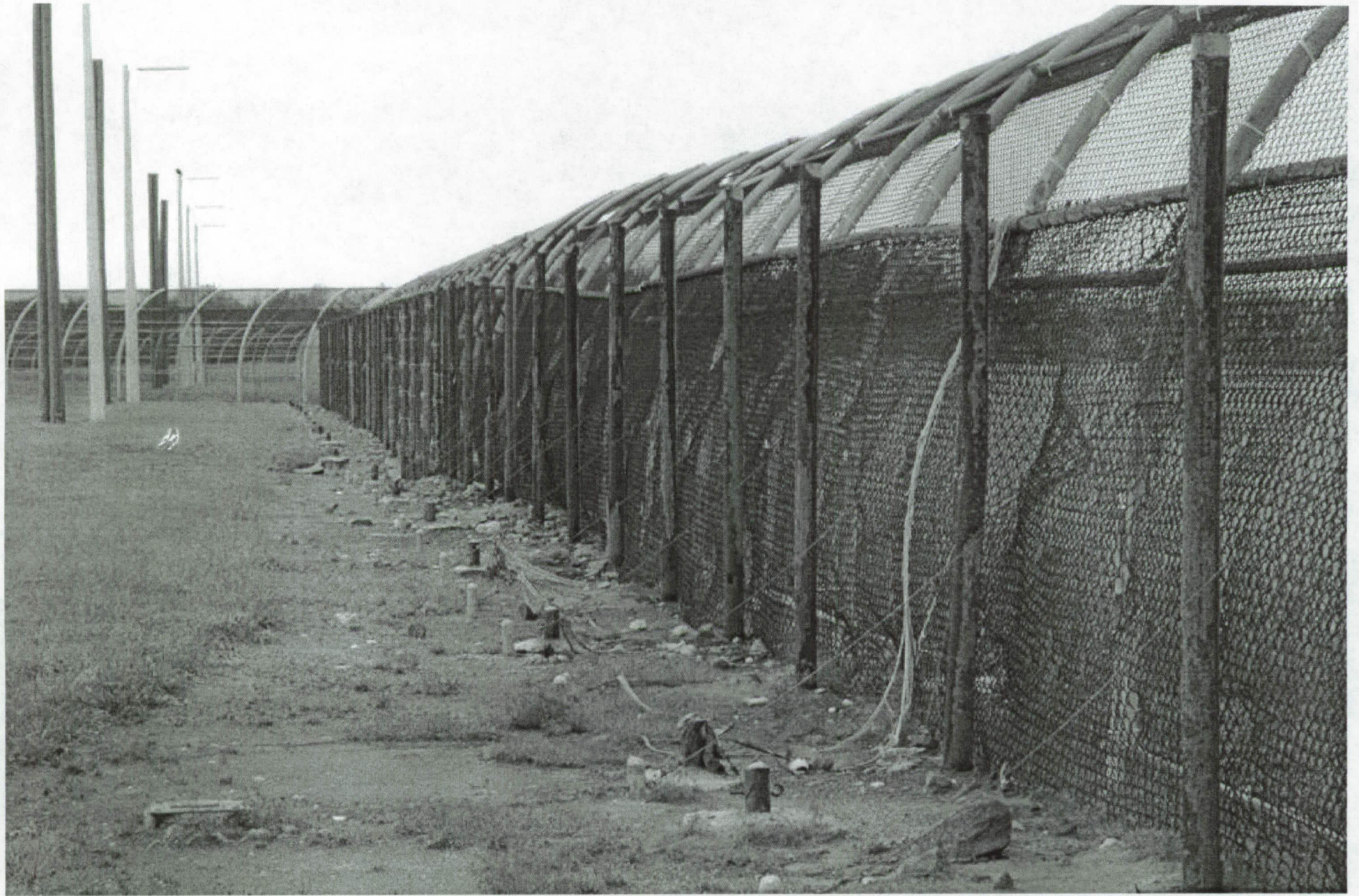
Damage to Pad perimeter fence from chunks of martite blown out of the flame trench
