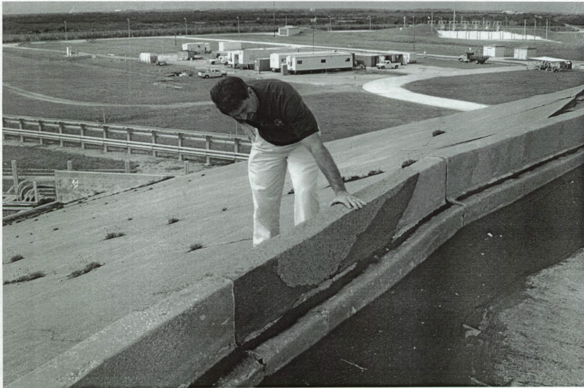
Damage to concrete wall due to FOD caught in the launch blast
