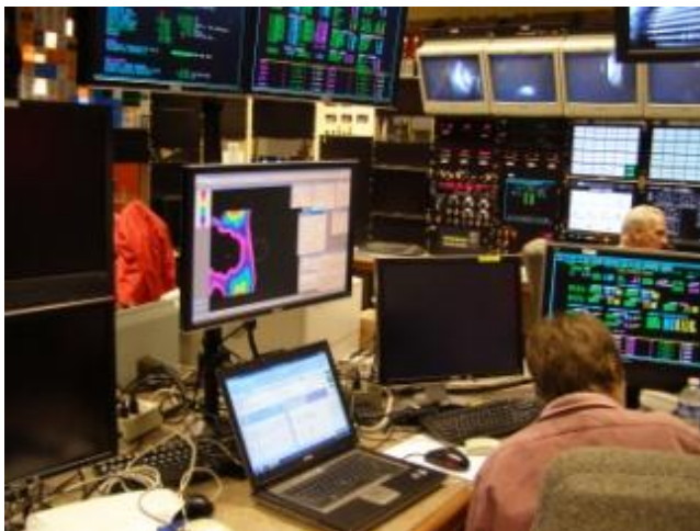
PSL Control Room
